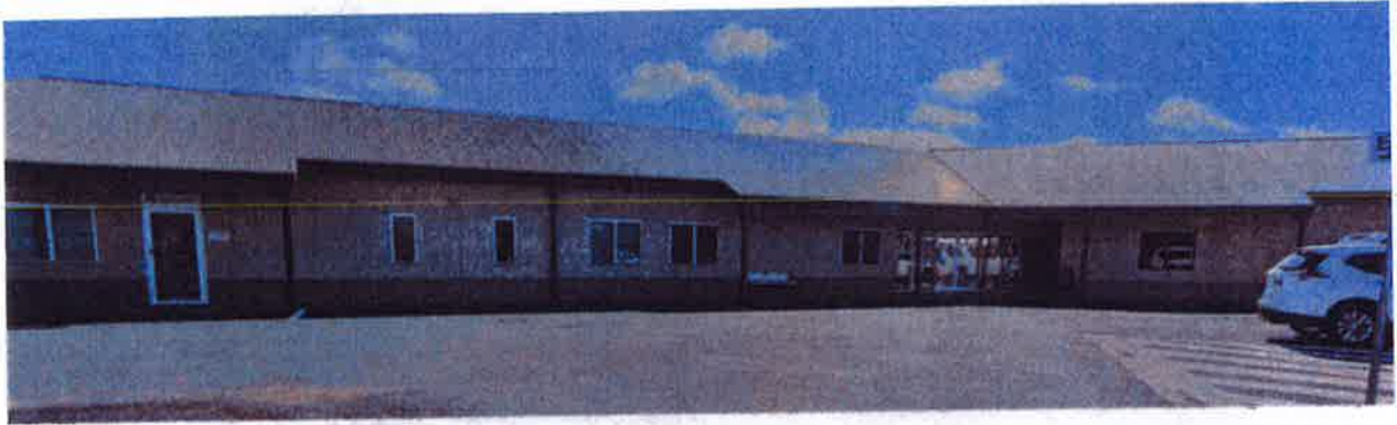
Building front: full re-paint of external walls.
